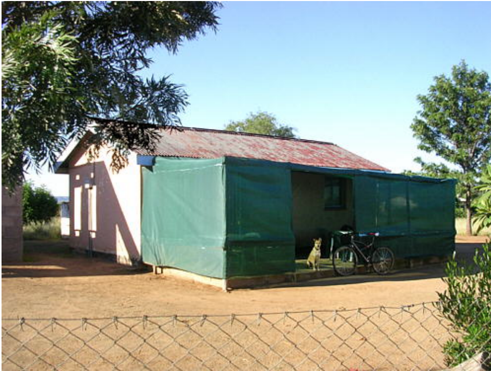
View of the northeast corner of the house and plot
